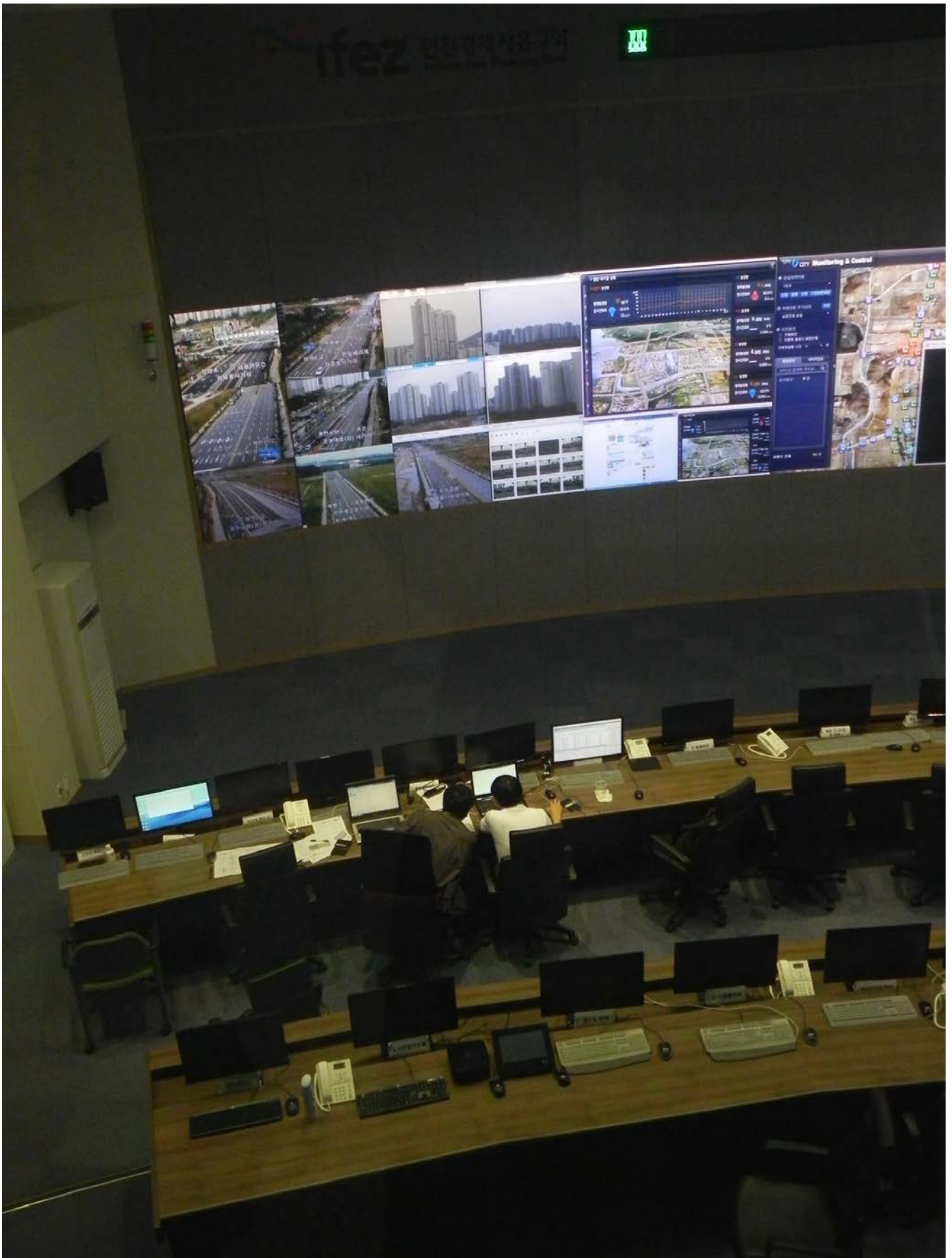
Figure 5. Songdo Control Room, September 2, 2013
